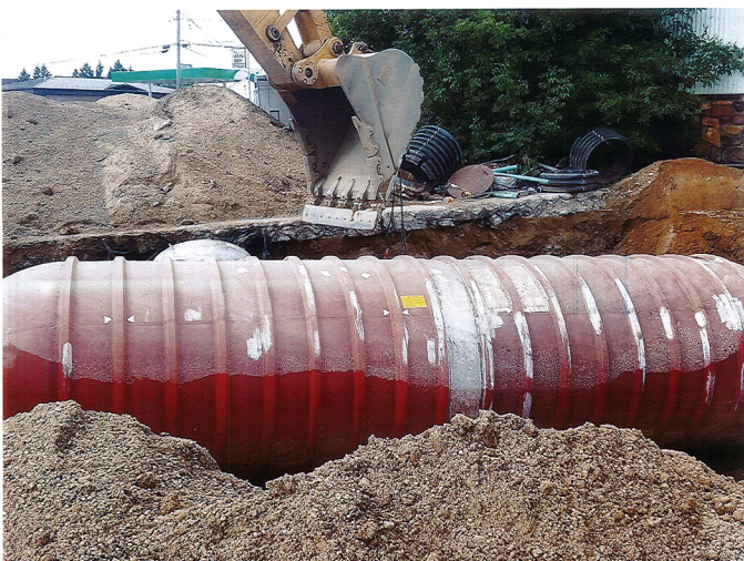
Figure 8: Tank Removal in Bovey
