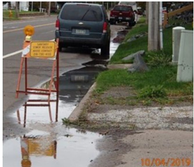
Above, untreated wastewater flows in the street of a Minnesota community in October 2019. In some locations, releases have entered not only streets, but also parks and yards, where residents, especially children, can inadvertently come into contact with wastewater.
