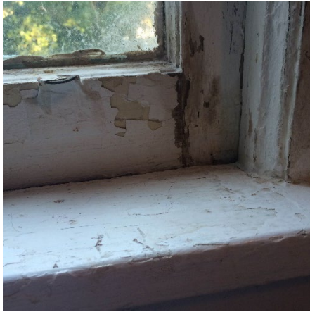
Chipped or peeling lead paint
