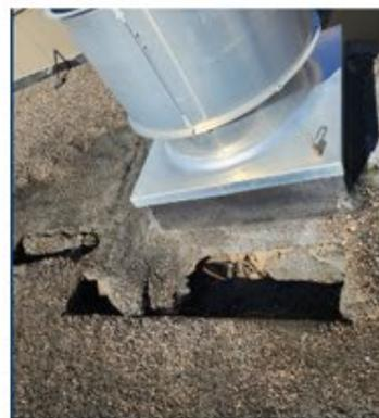
Hole in roof at Stillwater causing massive leaks
