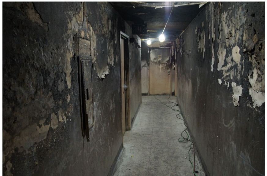
Figure 10: 14th story corridor (looking west from Apartment 1407)
