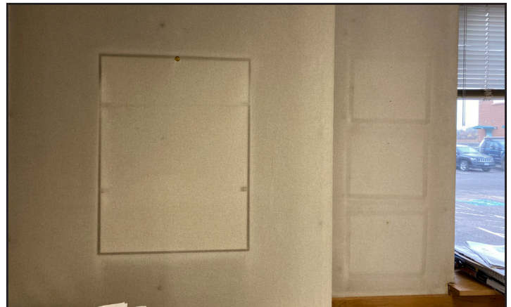
Heating and ventilation systems have reached their useful life, causing air quality and health concerns. The vents that do run are constantly cleaned and full of debris within a matter of days. Items have been removed from the walls and black outlines of the frames remain.
