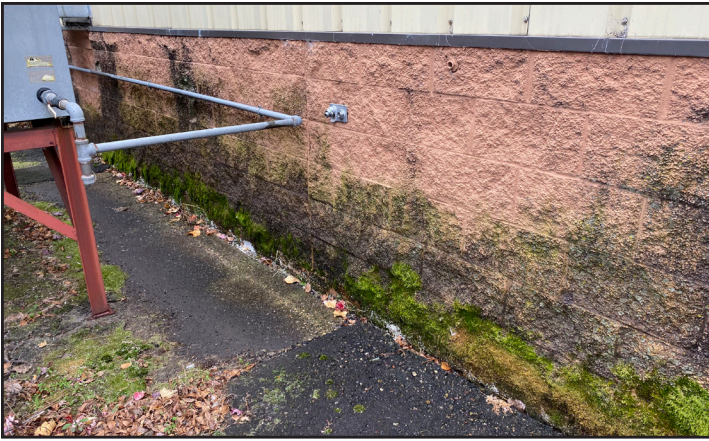
Mold is present on the exterior of the building due to moisture and drainage issues.
