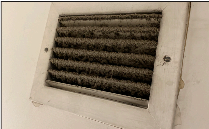
Heating and ventilation systems have reached their useful life, causing air quality and health concerns. The vents that do run are constantly cleaned and full of debris within a matter of days. Items have been removed from the walls and black outlines of the frames remain.
