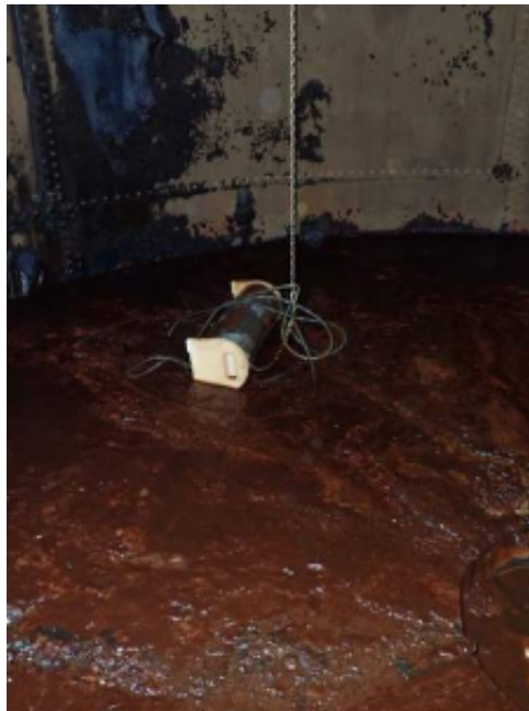
Condition of Water Tower from 2023 Inspection Report
