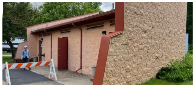
Current Lebanon Hills Restrooms Building
