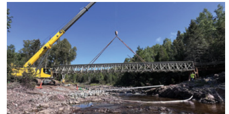
AFTER: Tettegouche State Park High Falls Bridge replaced, August 2025.
