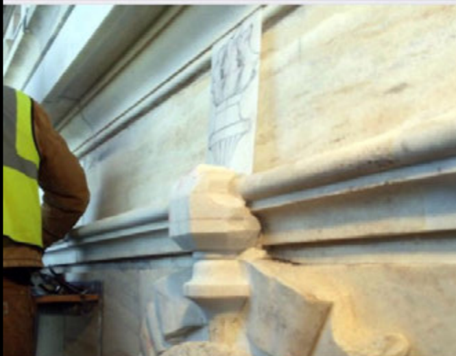
Then the sides of the torch are roughed out to give the flame its three-dimensional shape.
