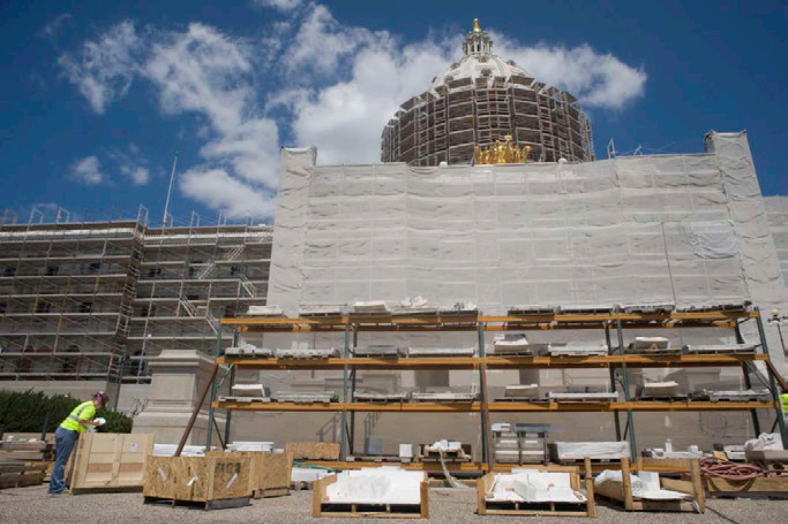
The new white marble arrived in crates and stored for its use on the Capitol.
