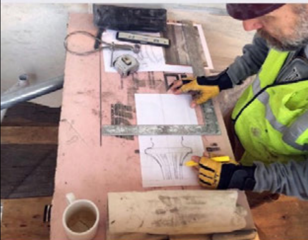
Templates are used extensively to help guide the process. Here, a master carver develops a historically-accurate template, using a photo from 1909 for the new torch.
