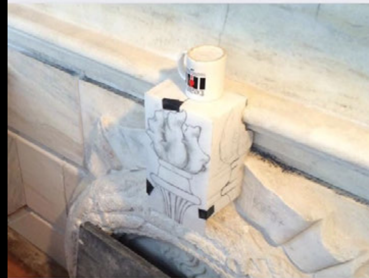
The template is taped to the marble block and used as a stencil.
