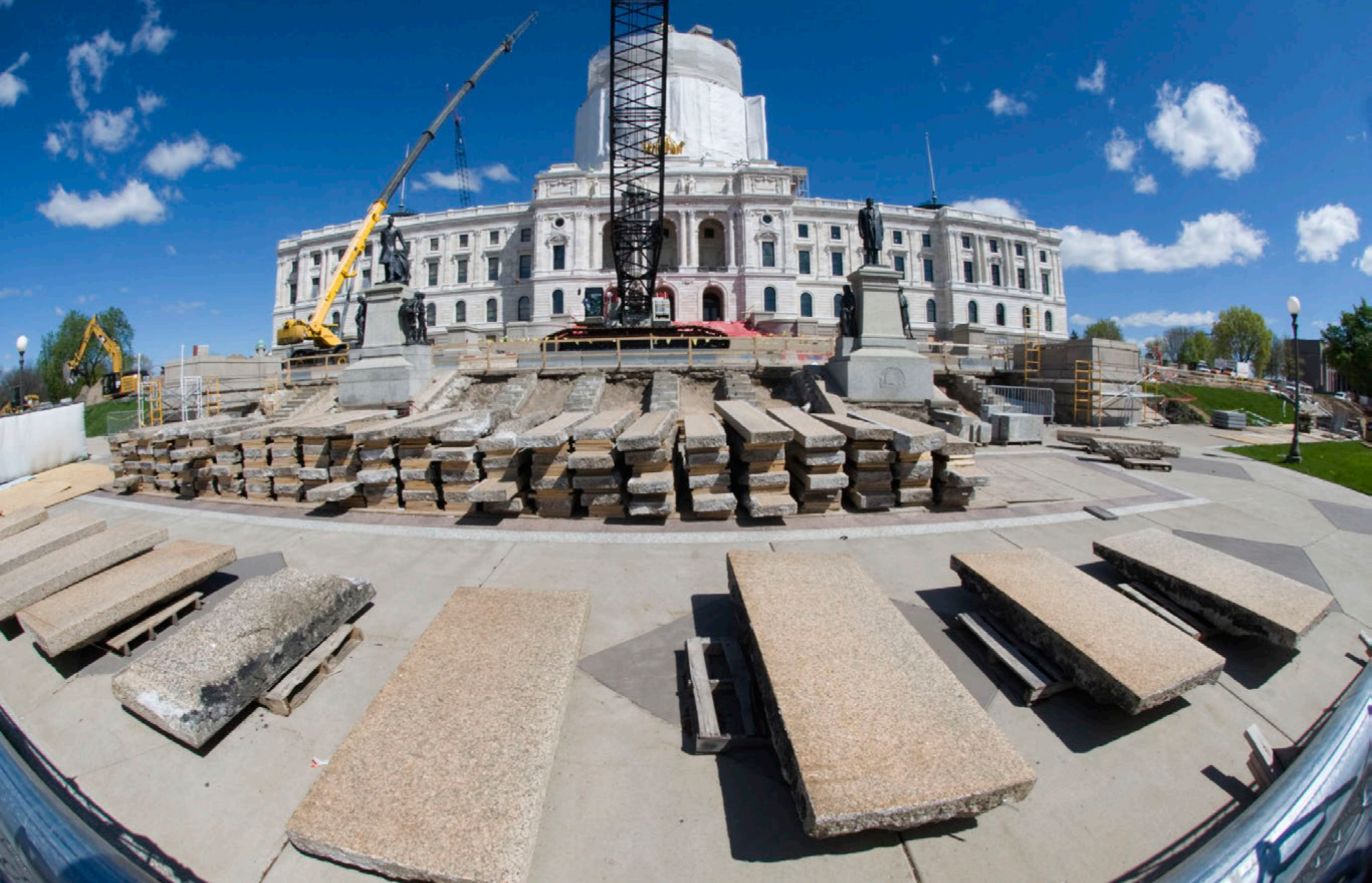
The Granite steps stacked in front of Capitol waiting for installation.
