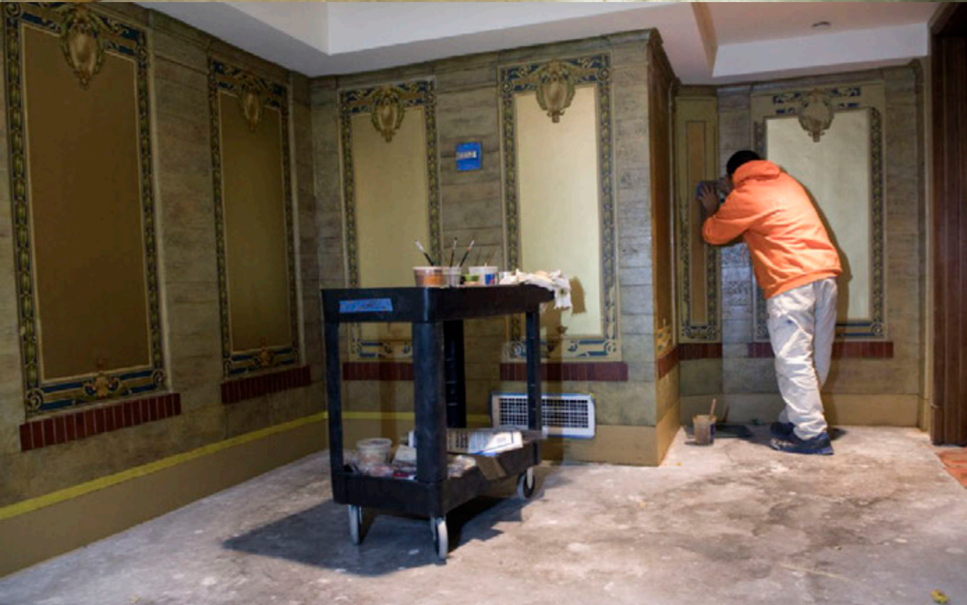
The Supreme Court Dining Room mural panels being restored. It had not been used for 60 years. It had extensive water damage.
