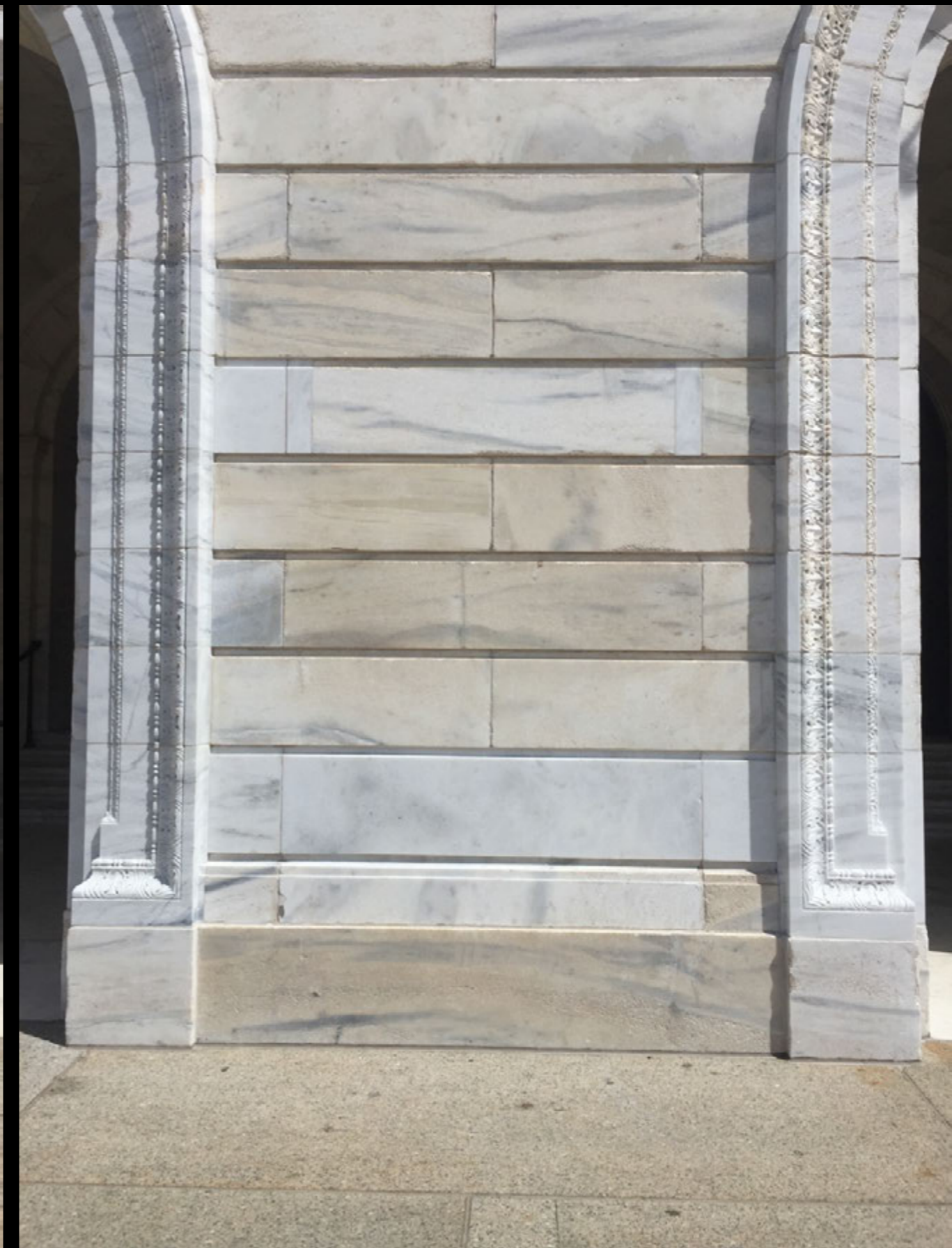
40% of the exterior white marble was replaced. Note the new white marble contrasts with the original darker marble. June 2017
