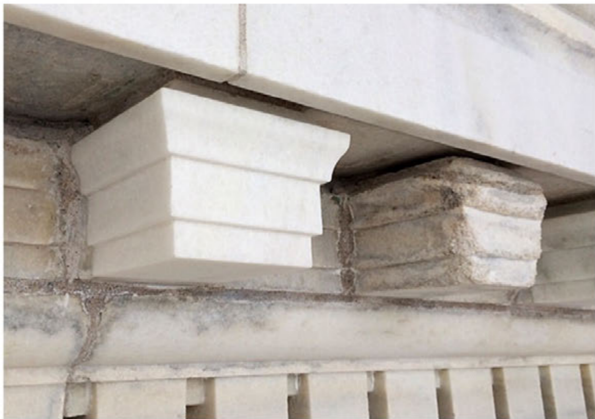
Courtesy of JE Dunn Construction
