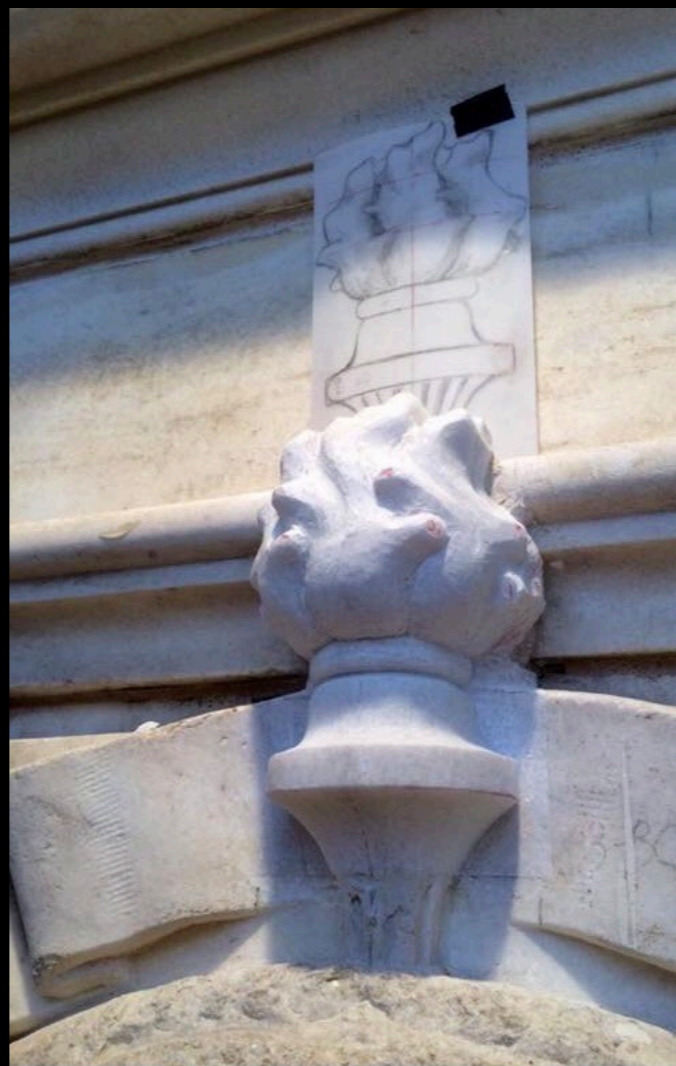
Small red points marked on the flame help guide final shaping and
