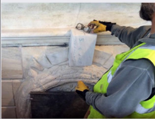
To begin the carving process, a plain block of marble is affixed to the exterior with stainless steel pins and epoxy.
