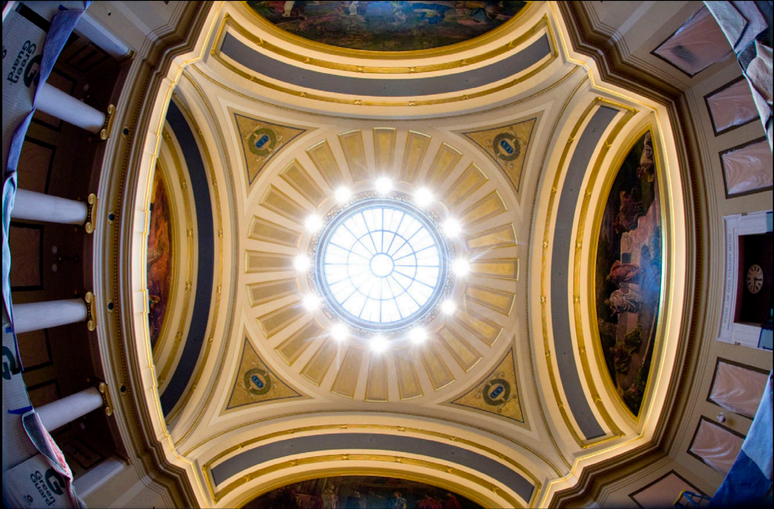
The restored Supreme Court Chamber skylight and interior dome.
