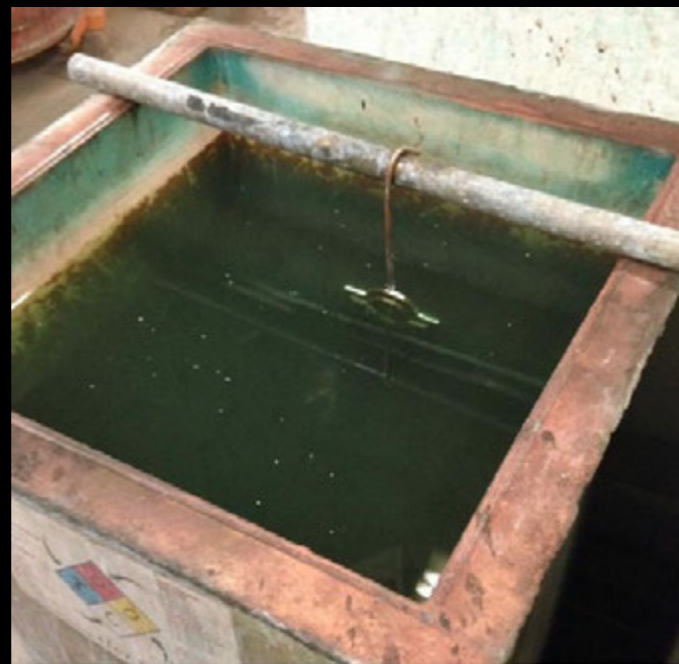
Next, the hardware was dipped into a solution to darken the metal finish to match the finish of the original hardware in the Capitol building.
