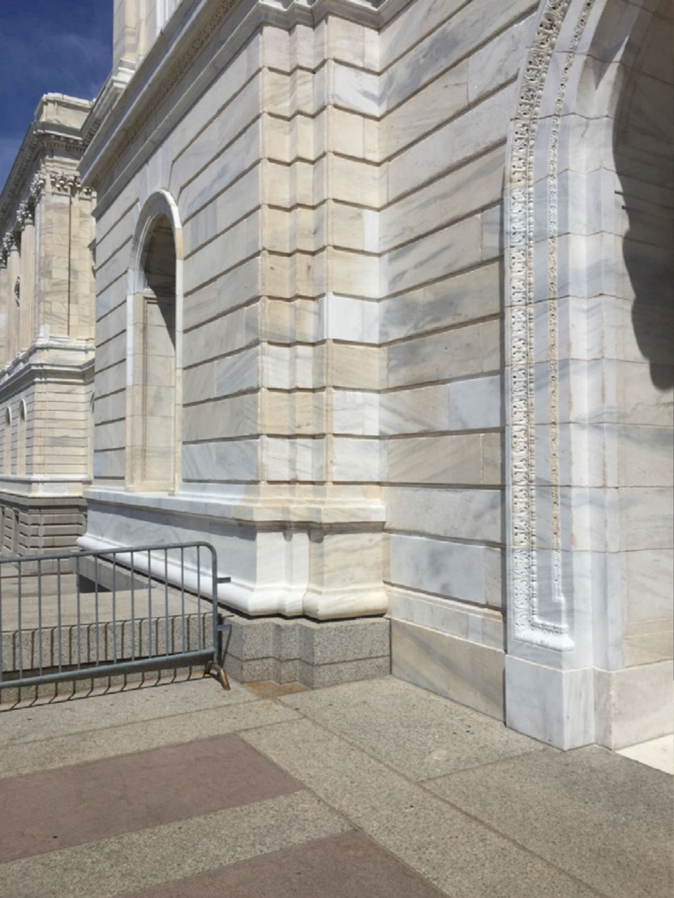
40% of the exterior white marble was replaced. Note the new white marble contrasts with the original darker marble. June 2017
