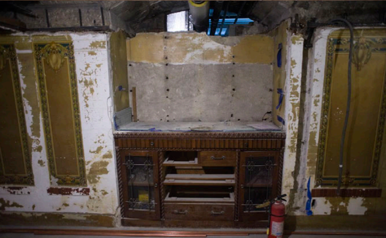
The Supreme Court Dining Room as it was found at the beginning of the restoration. It had extensive water damage. It had not been used for 60 years. The wooden China and silverware serving cabinet was in severe disrepair. The restored cabinet is ready for use at lower right.
