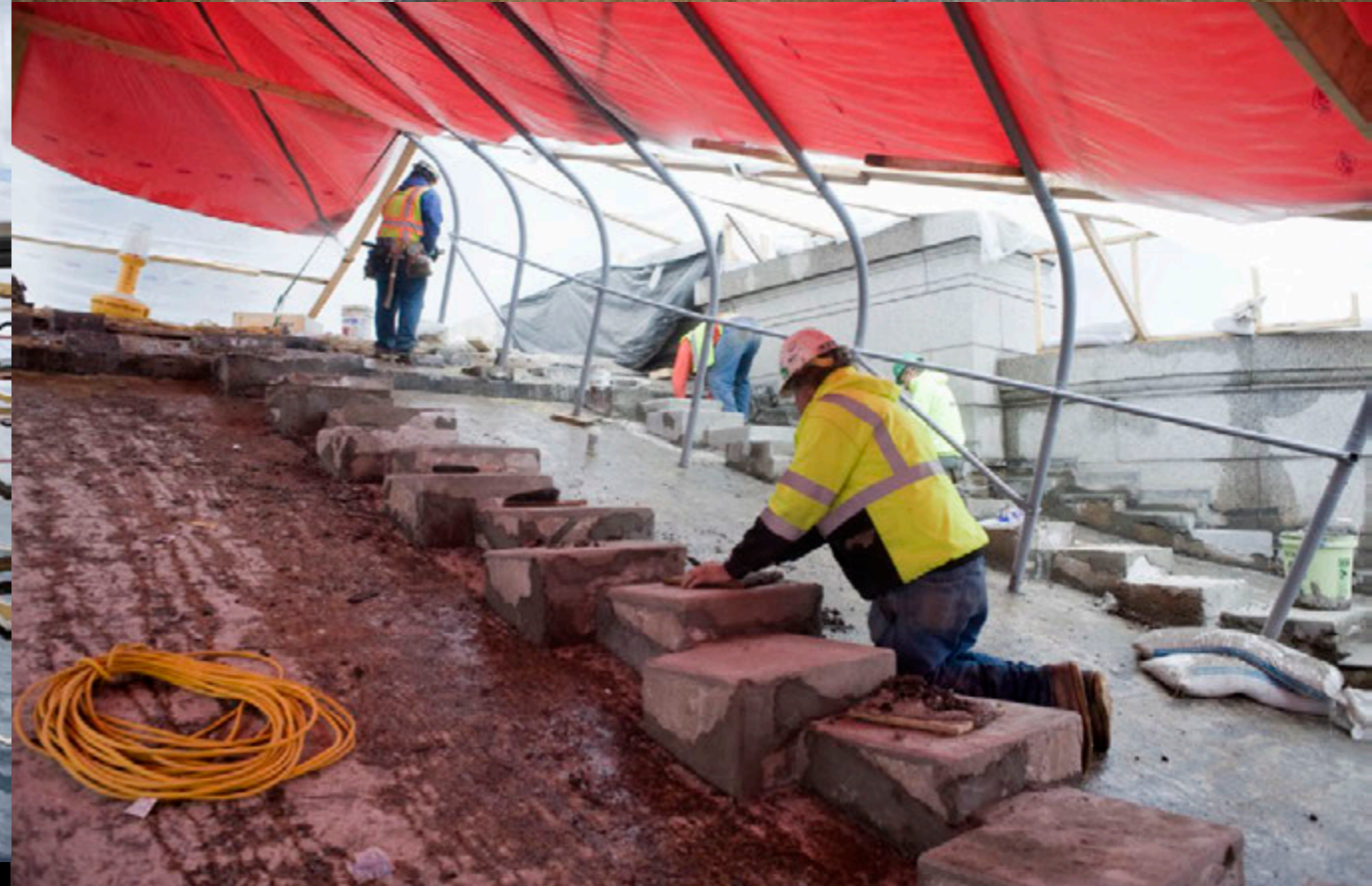
Granite steps in front of Capitol needed repairs, replacement and resetting. This was an additional $22 million cost that was discovered during the foundation restoration of the Capitol.
