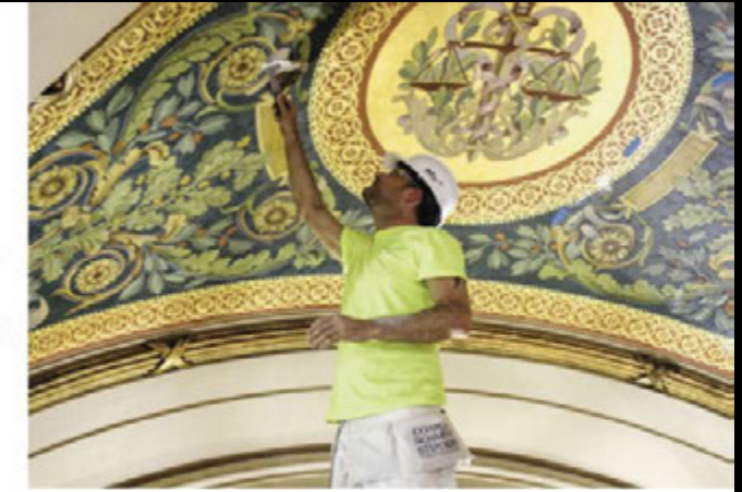
Restoring the intricate decorative artwork on the house chamber ceiling.
