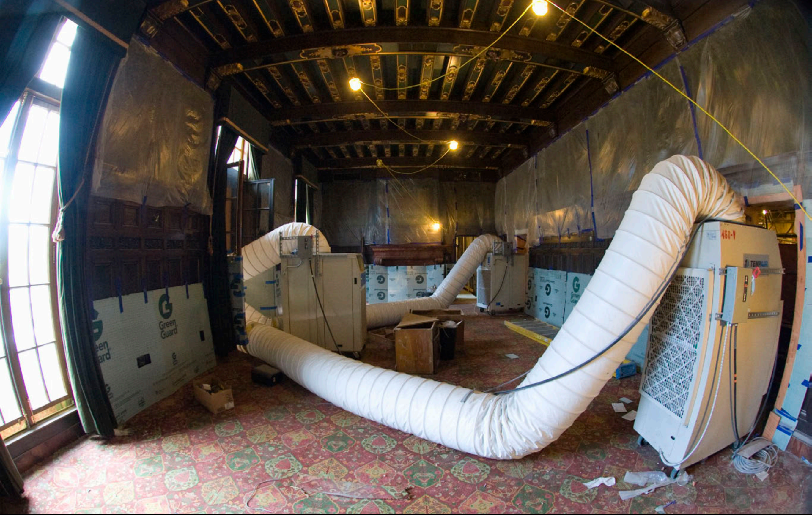
Minnesota House of Representatives Retiring Room being used to pump fresh air into the House Chamber during its Restoration.
