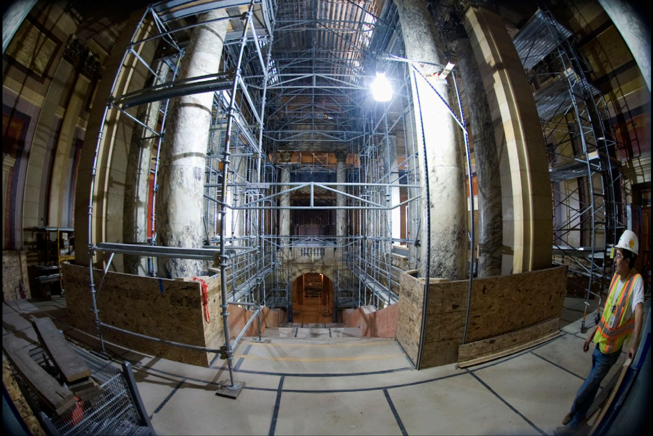
Scaffolding fills the East and West Grand Staircases.
