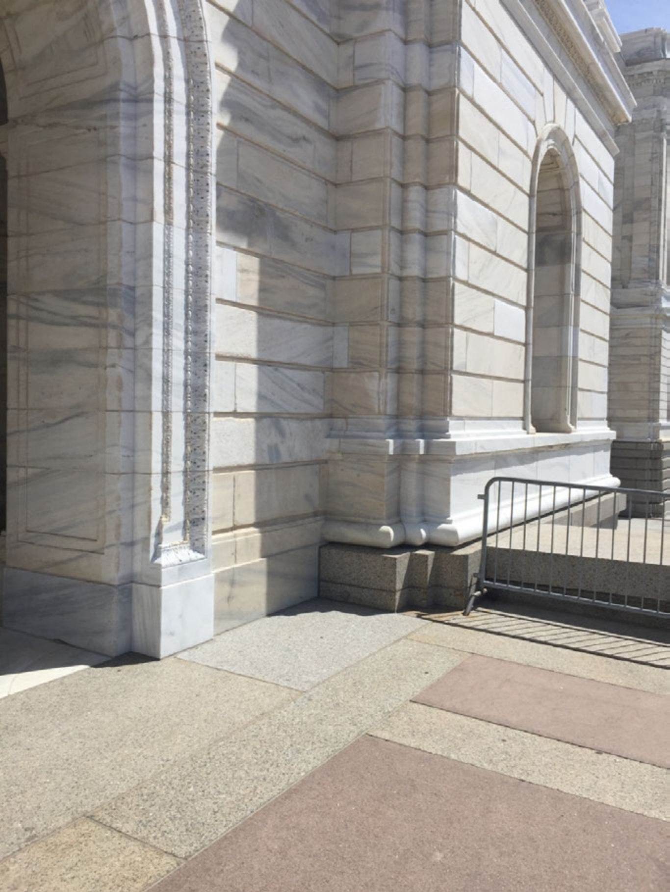
40% of the exterior white marble was replaced. Note the new white marble contrasts with the original darker marble. June 2017
