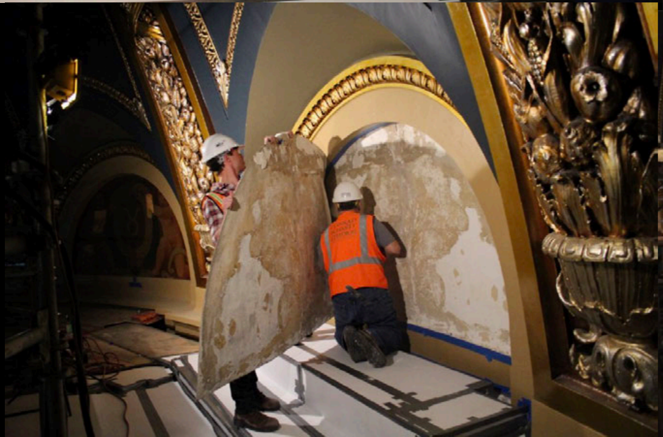
Using a long spatula, a conservator carefully begins separating lunettes shaped “zodiac” canvas mural from a wall in the Rotunda in order to repair the damaged and disintegrating plaster behind it.
