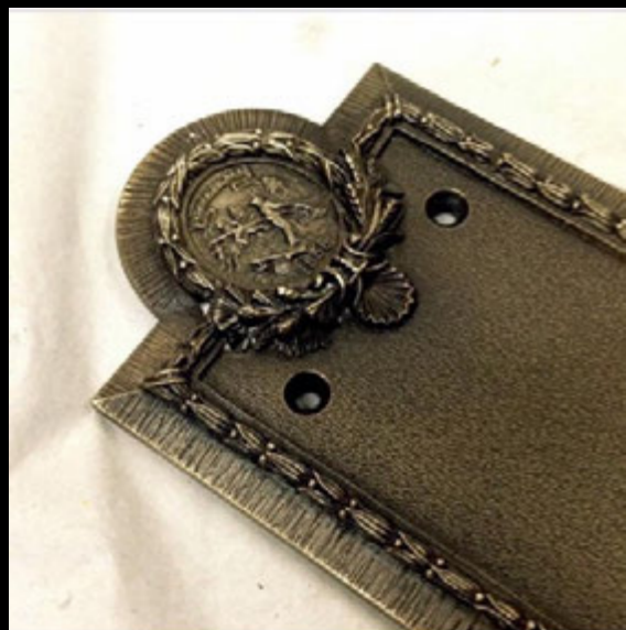
This piece of hardware is called an escutcheon. It is a flat piece of metal for protection and ornamentation around a keyhole, door handle, or light switch. The escutcheons in the Capitol feature the State of Minnesota seal used in the early 1900s.
