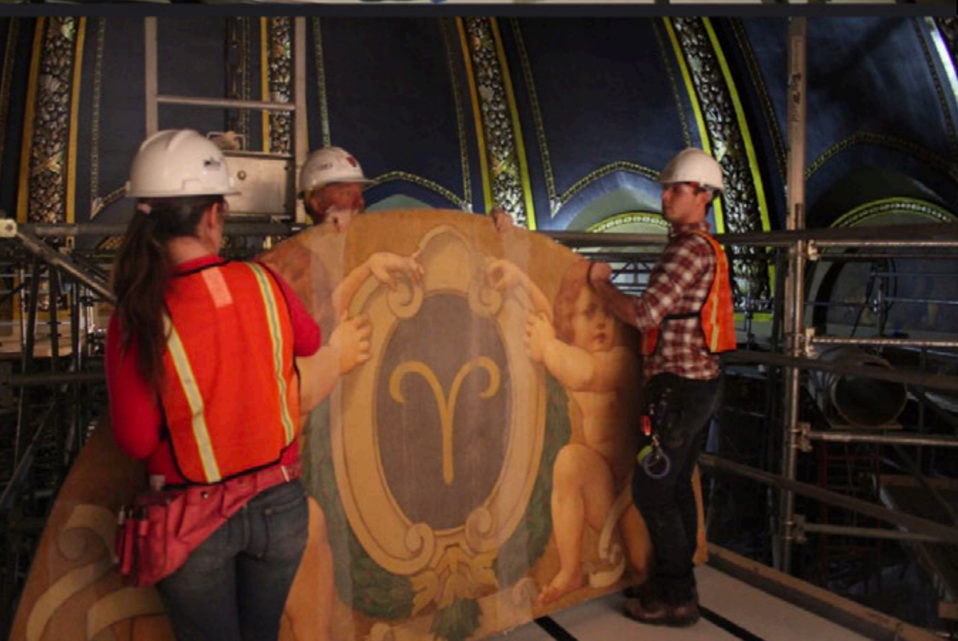
Using a long spatula, a conservator carefully begins separating lunettes shaped “zodiac” canvas mural from a wall in the Rotunda in order to repair the damaged and disintegrating plaster behind it.
