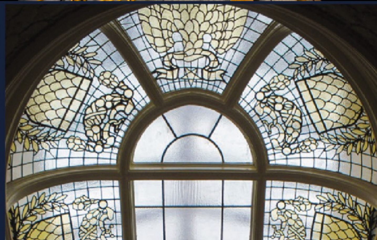
It was discovered the skylight was on the verge of collapsing and would have fallen down without structural repairs. Special conservation methods had to be used to preserve it.
