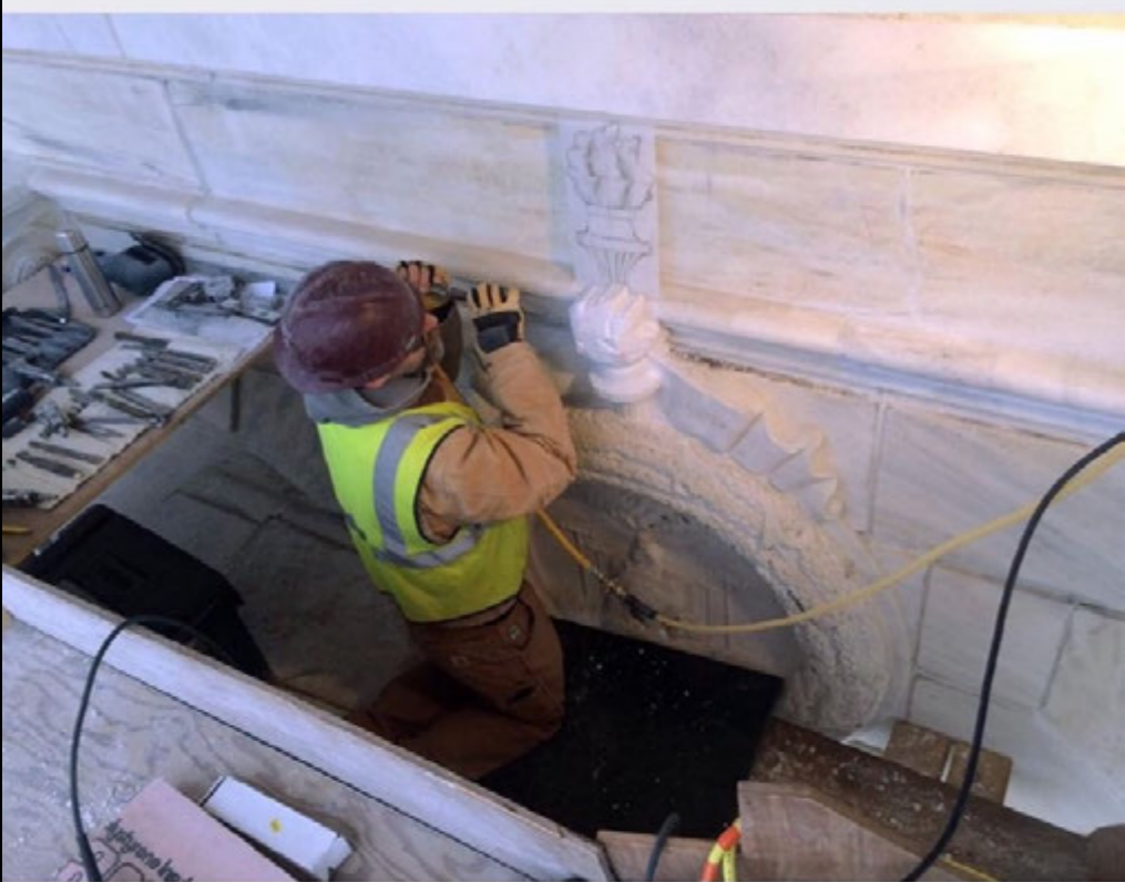
Next, the master carver sculpts more intricate detail, using tools essentially identical to those used during the Capitol's original construction in 1905.
