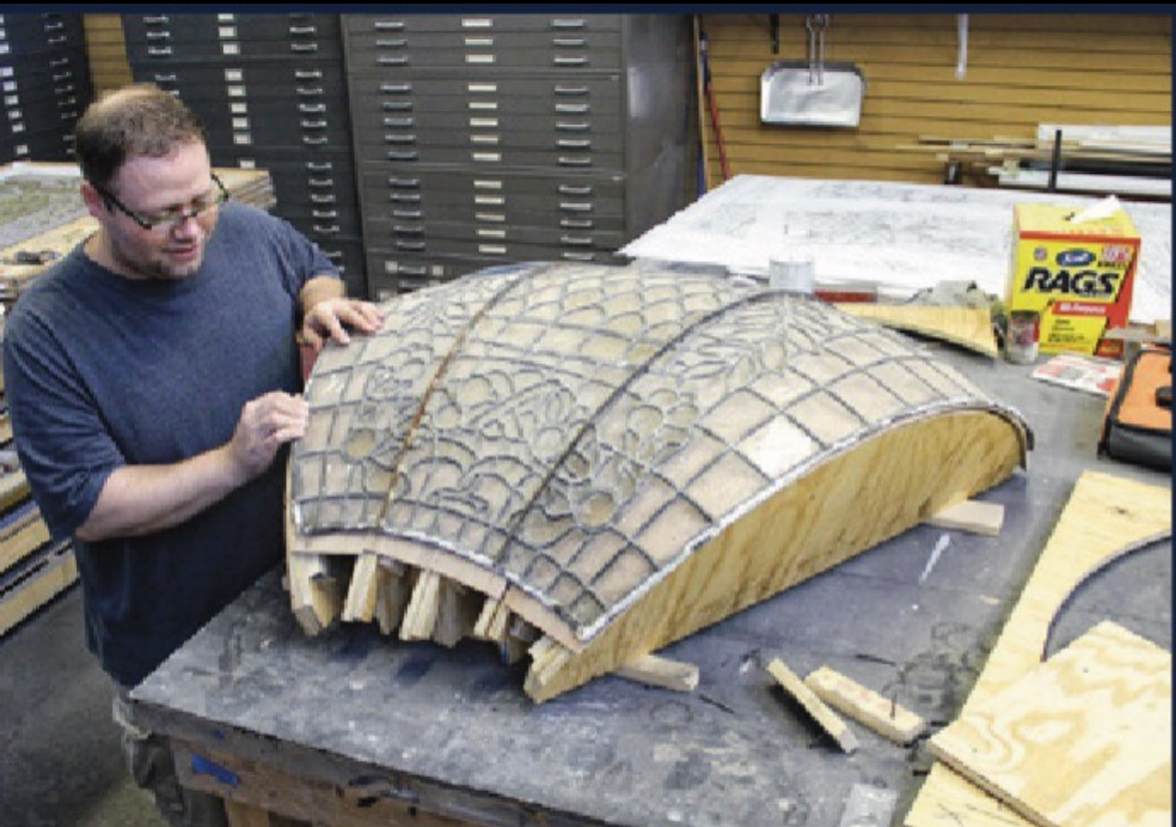
It was discovered the skylight was on the verge of collapsing and would have fallen down without structural repairs. Special conservation methods had to be used to preserve it.
