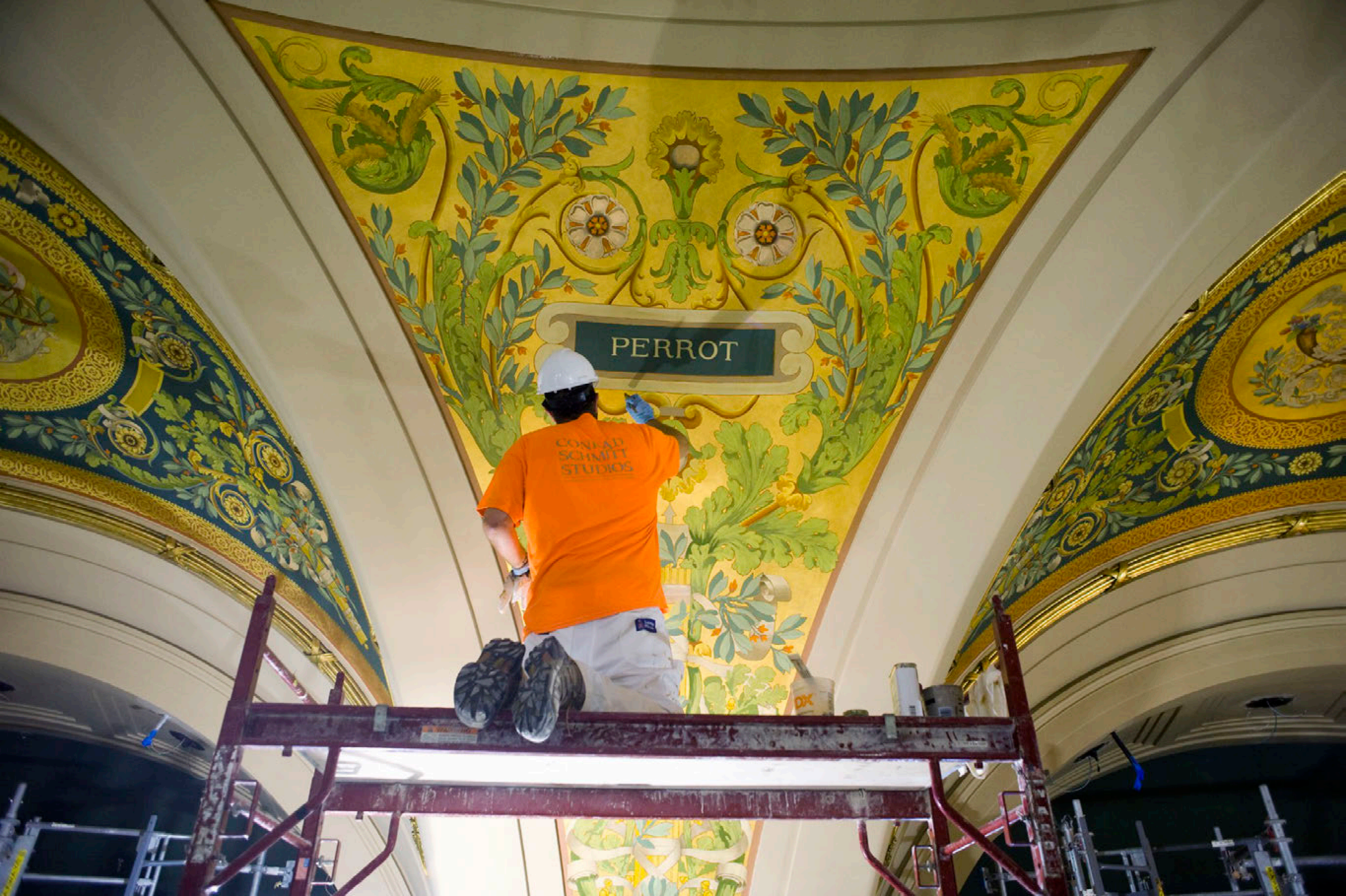
The House Chamber restoration of the painted areas of the ceiling.
