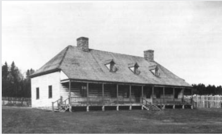
The Great Hall, reconstructed in 1974 on the basis of research into the design of the original building, is one of the attractions at Grand Portage National Monument.
