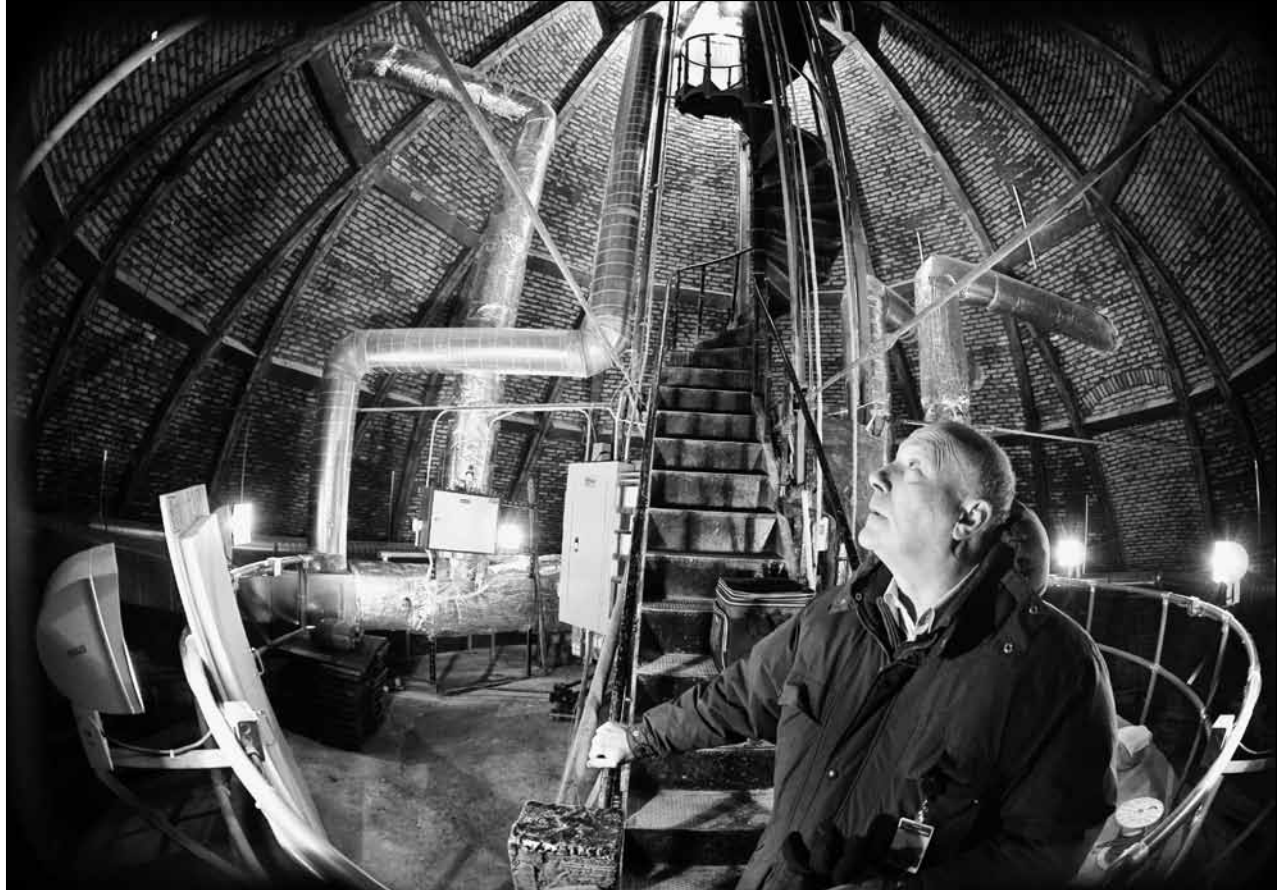
Harvey Jaeger, principal project coordinator of the Department of Administration's Real Estate and Construction Services Office, explains the air exchange system that has been installed between the interior and frost dome.
